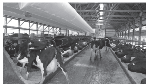
Positive pressure tube system to drive fast moving air into the lying area directly ~100 stall pen current maximum
